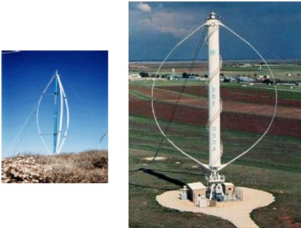
**FIGURE D-3 Examples of VAWTs (Left: FloWind Corporation VAWT at Tehachapi, California. Photo credit: R. Thresher. Source: Photo #04688, NREL 2004b. Right: Darrieus-design VAWT operated as a wind energy technology test bed by Sandia National Laboratories at the U.S. Department of Agriculture research station at Bushland, Texas; 138 ft (42 m) high, 112 ft (34 m) in diameter. Photo credit: Sandia National Laboratories. Source: Photo #01671, NREL 2004b.)**
