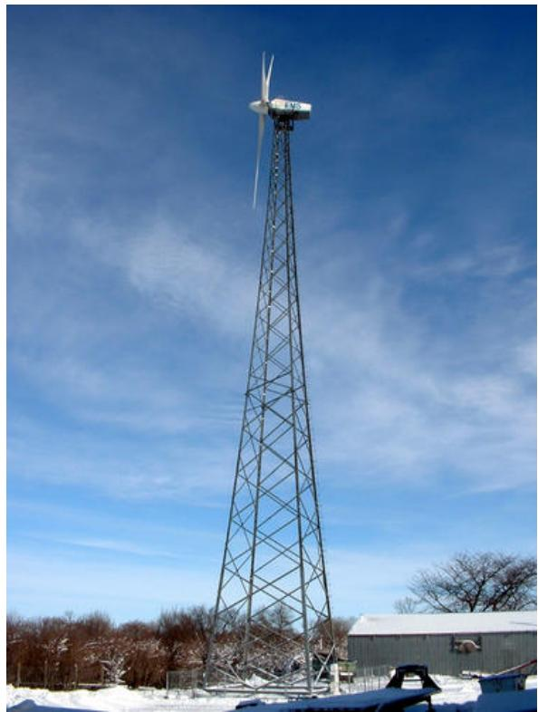
**FIGURE D-8 Lattice-Type Wind Turbine Tower in South Dakota (A Vestas Model V17 wind turbine mounted on a lattice-type tower in Gary, South Dakota. Photo credit: Energy Maintenance Service, Inc., Sept. 1, 2002. Source: Photo # 12449, NREL 2004b.)**
