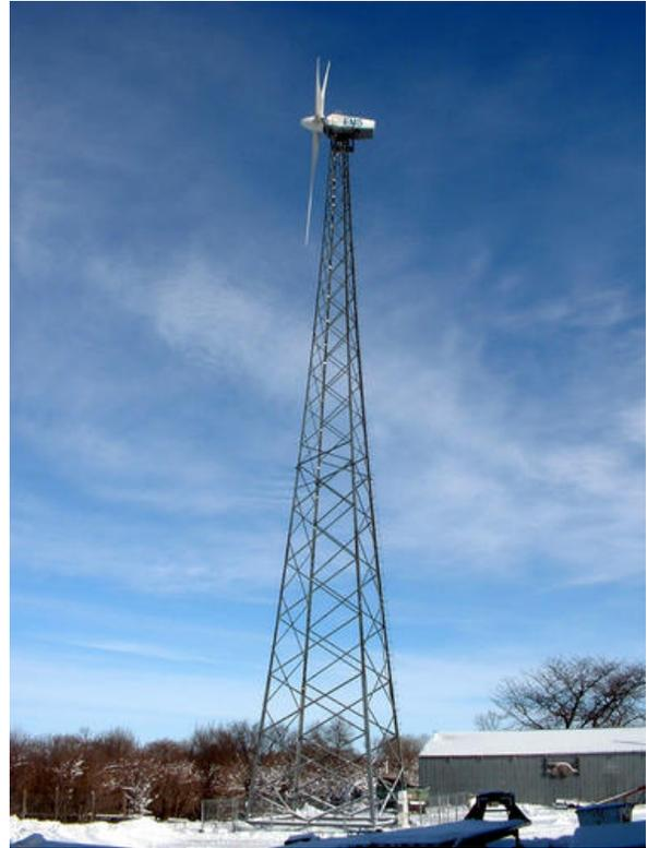
**FIGURE D-8 Lattice-Type Wind Turbine Tower in South Dakota (A Vestas Model V17 wind turbine mounted on a lattice-type tower in Gary, South Dakota. Photo credit: Energy Maintenance Service, Inc., Sept. 1, 2002. Source: Photo # 12449, NREL 2004b.)**
