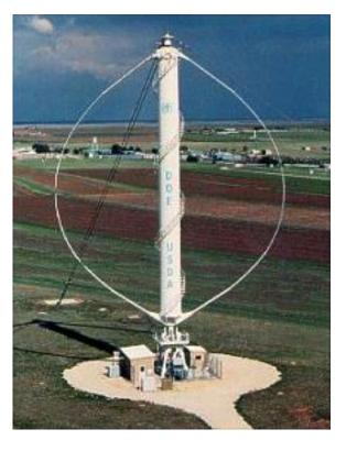
FIGURE D-3 Examples of VAWTs (Left: FloWind Corporation VAWT at Tehachapi, California. Photo credit: R. Thresher. Source: Photo #04688, NREL 2004b. Right: Darrieus-design VAWT operated as a wind energy technology test bed by Sandia National Laboratories at the U.S. Department of Agriculture research station at Bushland, Texas; 138 ft (42 m) high, 112 ft (34 m) in diameter. Photo credit: Sandia National Laboratories. Source: Photo #01671, NREL 2004b.)
